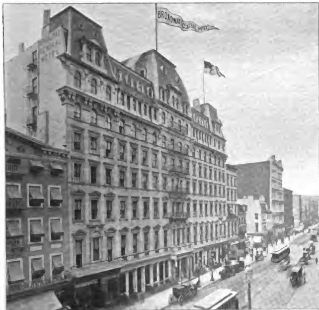
BROADWAY CENTRAL HOTEL, BROADWAY, OPPOSITE BOND STREET.
